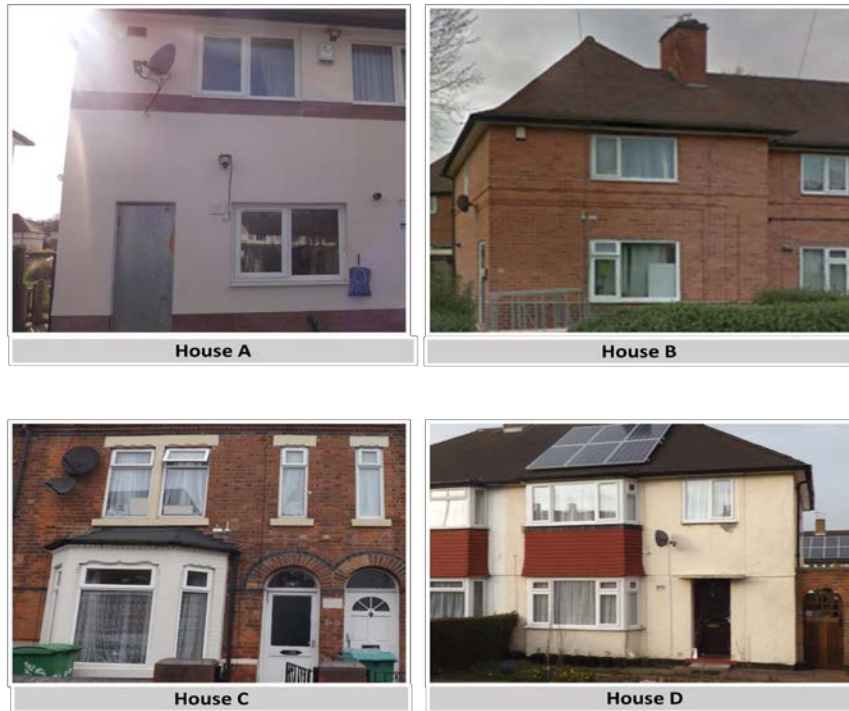
Fig 4. the four houses covered in this study.
