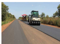
Construction of the Baoundaiali-Tengrela road
