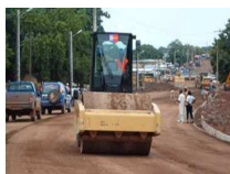
Construction of Abobo-Anyama Road
