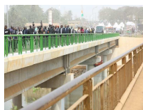
Construction of Bridge over the Marahoué
